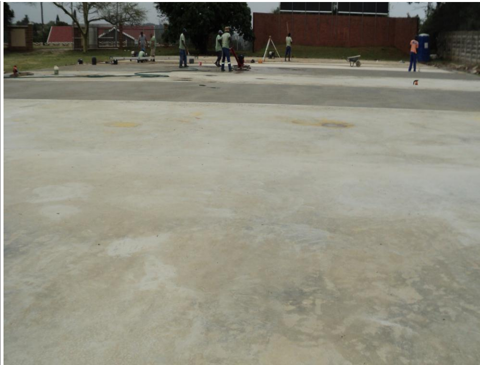
Slab after FRC Repair
